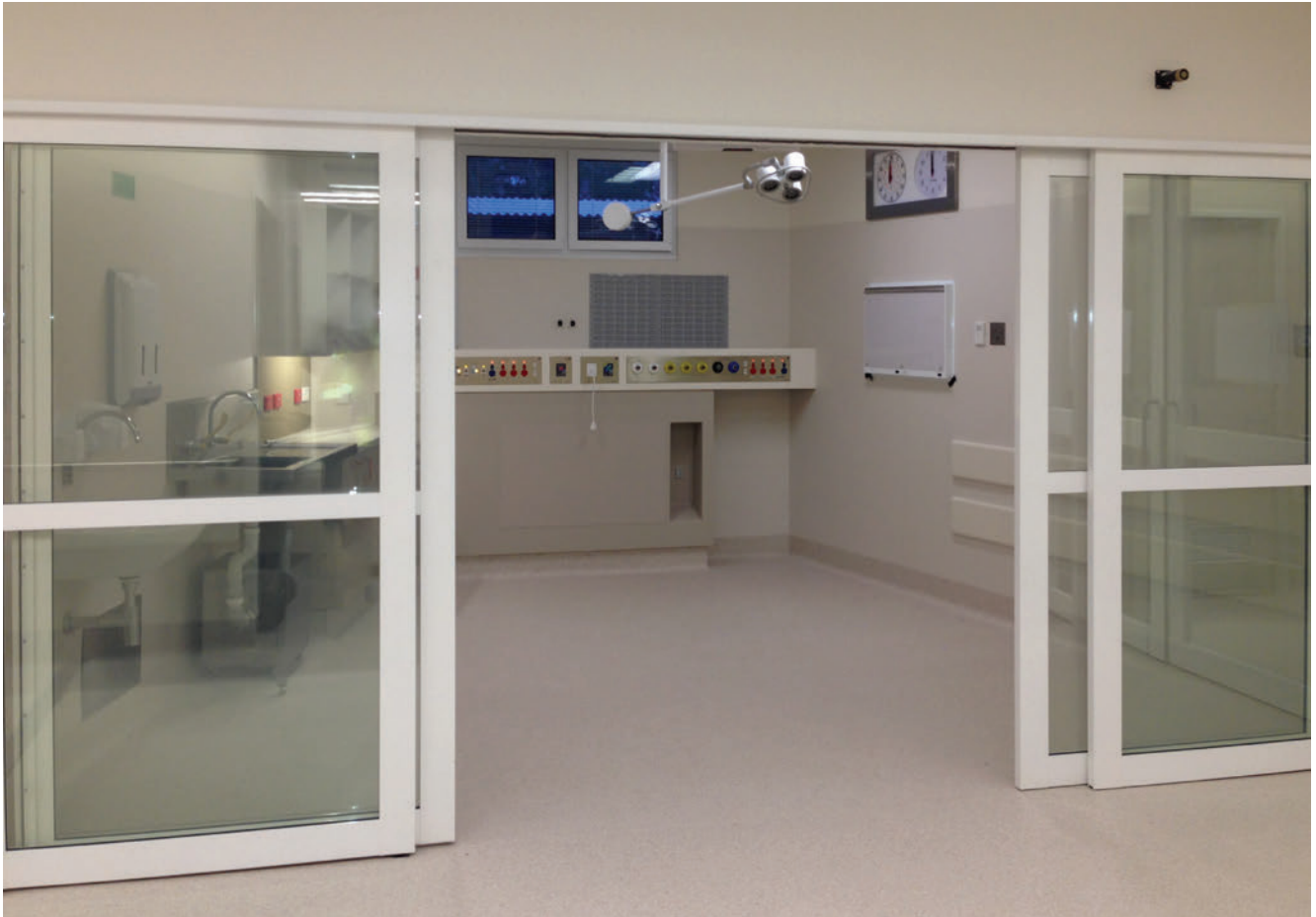
CS NewYorker doors with Switchable iGlass on CS ElecTrack - Fixed/Slide configuration
