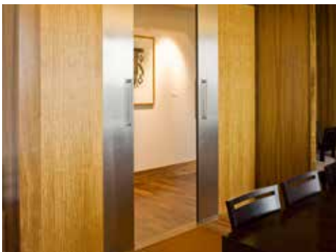
Bi-Parting unit with STC 42 / RW 42 dB doors incorporating magnetic joining seals
