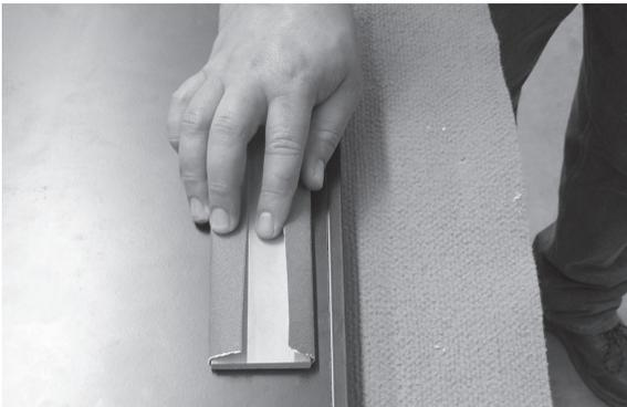
After sanding, follow with a thorough clean using methylated spirits to remove all dust and contaminants.
